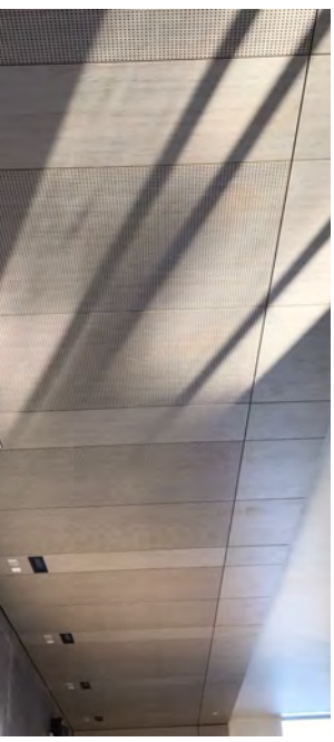
IMPACT PANELS AFTER INSTALLATION
