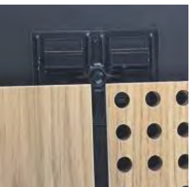
AT THE CORNERS THE CLIPS SHOULD BE MOUNTED VERTICALLY TO CAPTURE THE BOARD YOU ARE FIXING AND THE NEXT. THE SCREWS SHOULD BE BLACK SO AS TO APPEAR INVISIBLE ONCE FIXED THROUGH THE CLIPS.
