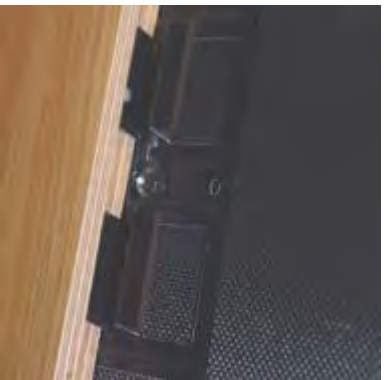
THE PANELS ARE FIXED USING THE SECRET CLIPS WHICH ARE TO BE PLACED INTO THE PRE-ROUTED EDGES TO LEAVE THE APPEARANCE OF A FIXTURE FREE INSTALLATION.
