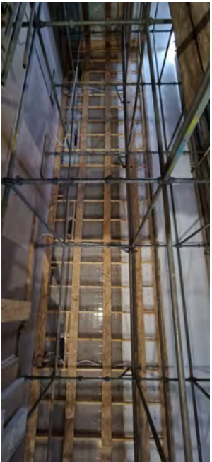
TIMBER FRAMEWORK BEFORE INSTALLATION OF IMPACT PANELS
